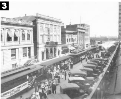
Looking southeast on Pierce between 3 rd and 4 th Streets
